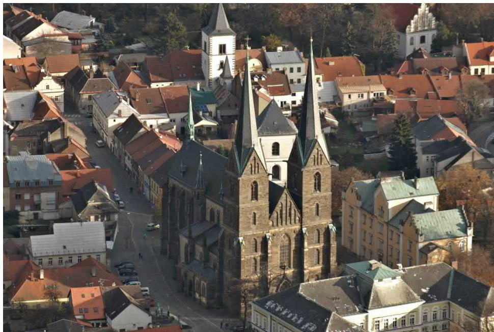
Fig. 34 Vysoké Mýto, Church of St. Lawrence in an oblique aerial photograph, view from the north-west; Martin Gojda 2020
