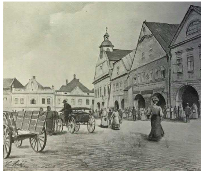
Fig. 9 Dvůr Králové nad Labem, T. G. Masaryk Square (view from the east), northern front of a built-up area with Renaissance building of the old town and burgher houses with arcades; Josef Král 1908
